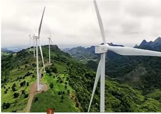
Figure 2. Sidrap Wind Turbine with a capacity of 75 MW
